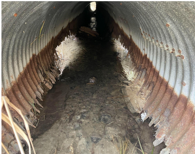
Image: Current undersized culvert on County Rd. 40.
