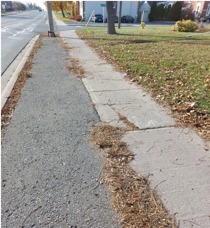
Image: Deteriorated sidewalk and asphalt.
