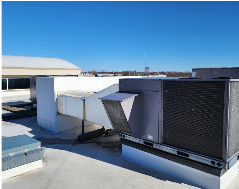
Image: Deteriorating exterior ductwork
