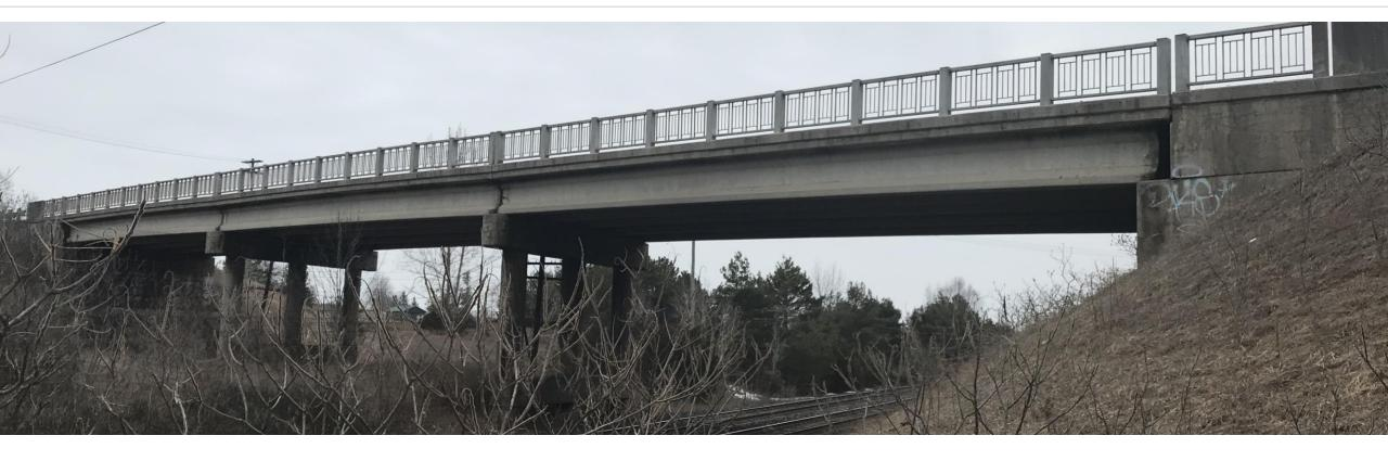
The Wooler Road CNR/CPR Overpass is in a state of deterioration and requires rehabilitation or replacement. The existing bridge is currently carrying two lanes, with no ability to widen to four lanes, and no capacity for active transportation facilities. Therefore, the City of Quinte West has the opportunity to identify and evaluate alternative solutions and determine a preferred bridge solution in accordance with the MCEA Process.
